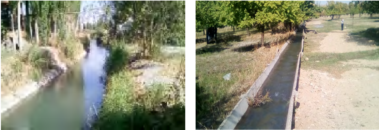
Figure 3. View of the concrete covered part of the Ak-Tatyr canal – the intra-farm part of the canal (left photo) and view of the tray section of the Jaiylma canal (right photo)
