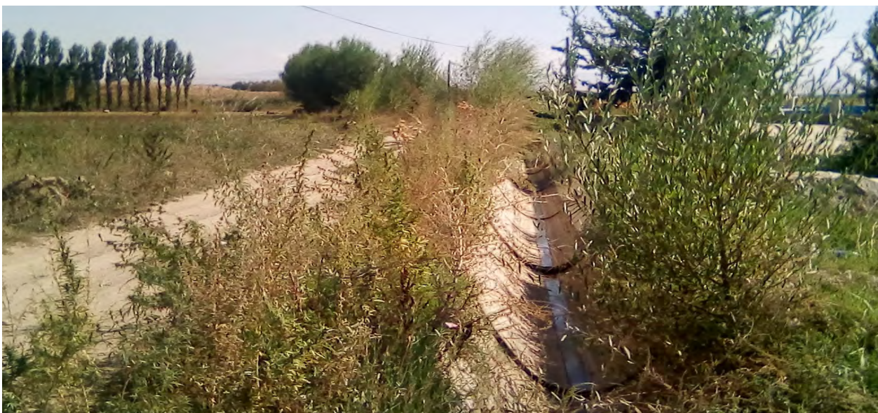
Figure 4. View of the rehabilitated part of the 1-2 Maya canal by reinforced concrete trays
