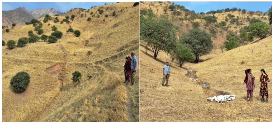
Figure 15: Gully plugging and check damming sites visited
