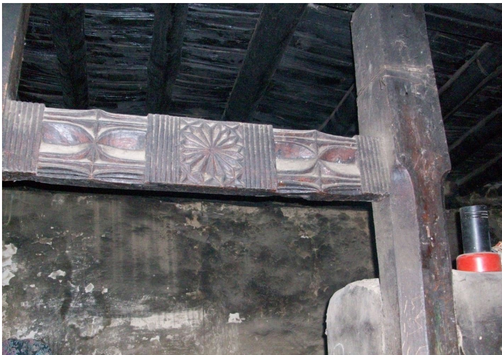
Photo 8 and 9: Bučkiĵj – the beam between the two columns in a traditional Pamirian house (the second photo was captured in a new-structure house, the first one – in an old-structure house).
